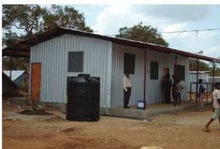
Constructing temporary shelters in Vavuniya
